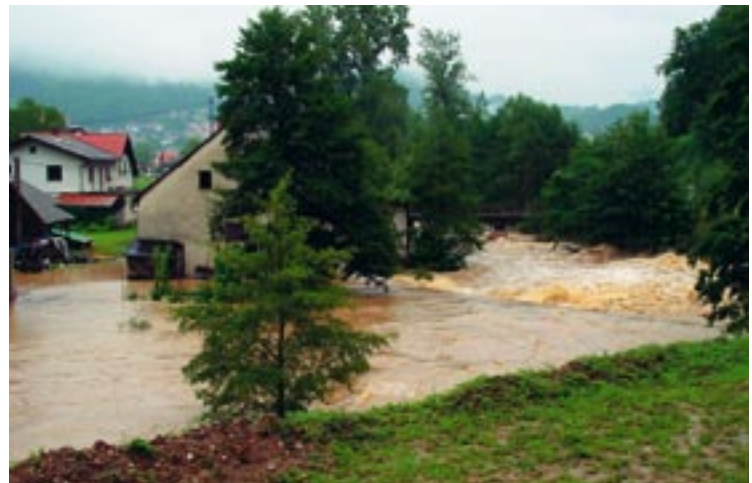
River Mirna flooded Boštanj, August 2005.
